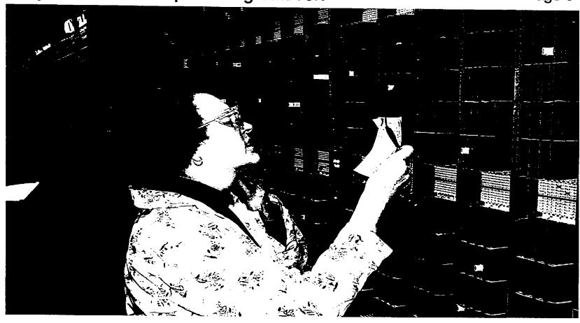
Step 6: Technician walks along Main Distributing Frame to locate both ends of jumper to be cut.
