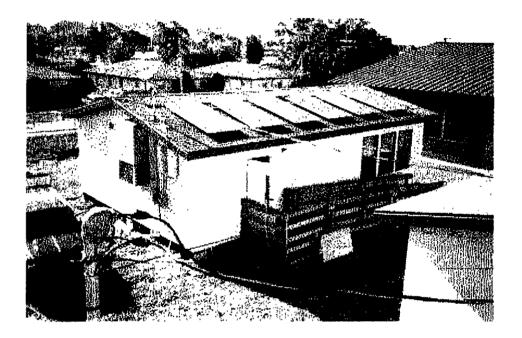
Figure 4-2 Portable Classroom Topped by PV Panels
