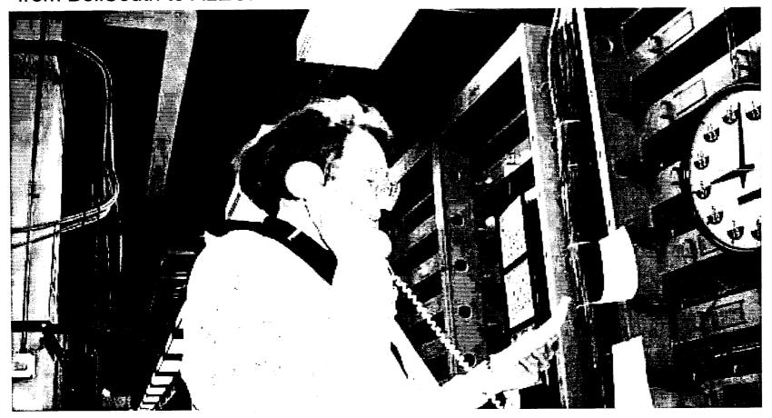
Step 5: Technician conducts ANAC test to verify that correct loop is being cutover.
