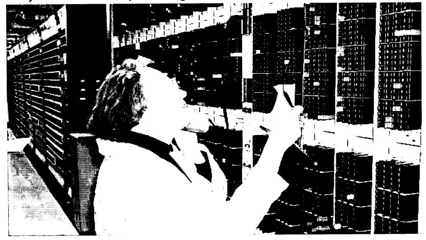
Step 6: Technician walks along Main Distributing Frame to locate both ends of jumper to be cut.
