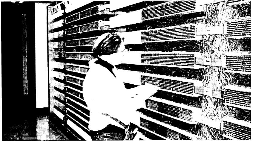
Step 8: Technician locates and removes end of jumper connected to the BellSouth cable pair.
