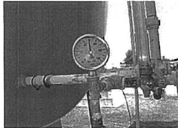
*Static distribution system pressure, 49 psi, (no pumps running.)*
