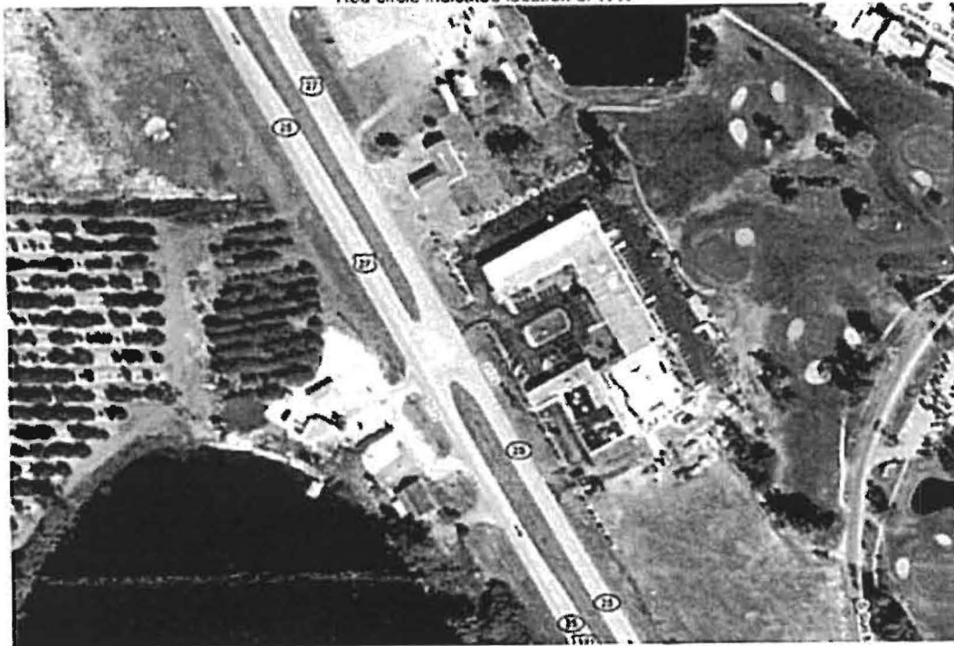
Red circle indicated location of WTP
