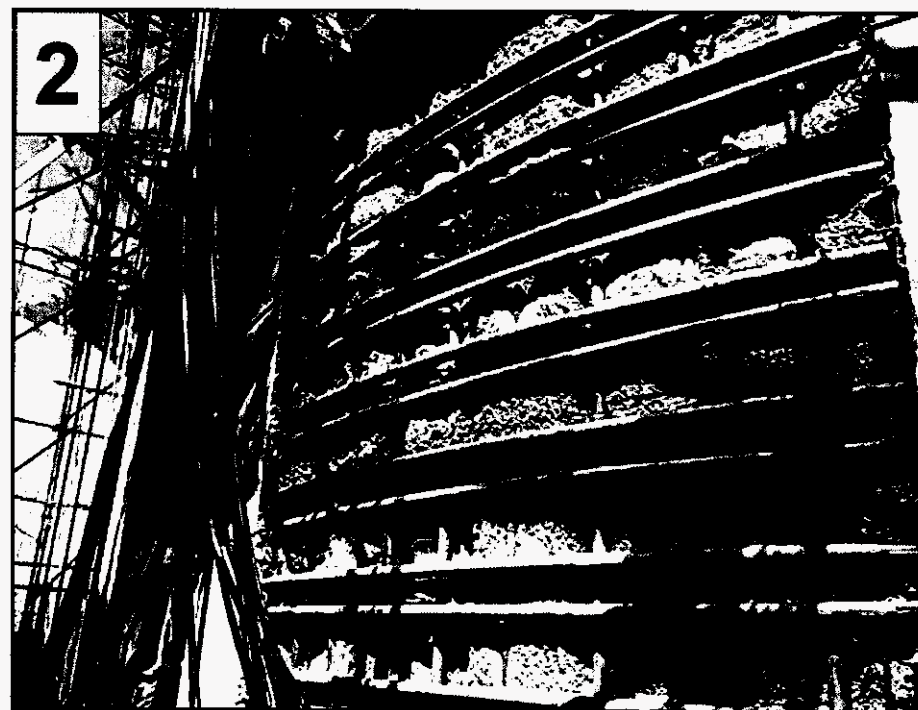
Tendon Sleeves Exposed
