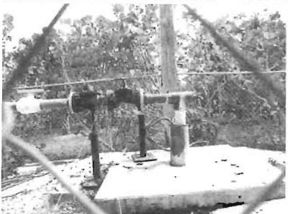
Well #1 need to repair the pad
