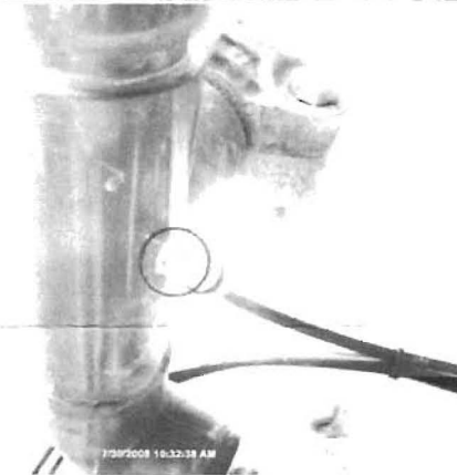
Leaking at RO reject outlet
