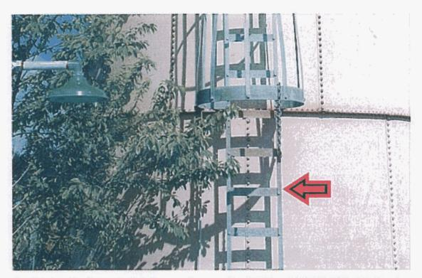
Shell ladder in above photo is in compliance with OSHA and AWWA D100-96, Section 7.4: Ladders, 7.4.1: Outside Tank Ladder, regulations. We recommend installing a cable type ladder safety device, and posting a Fall Protection Required sign.
