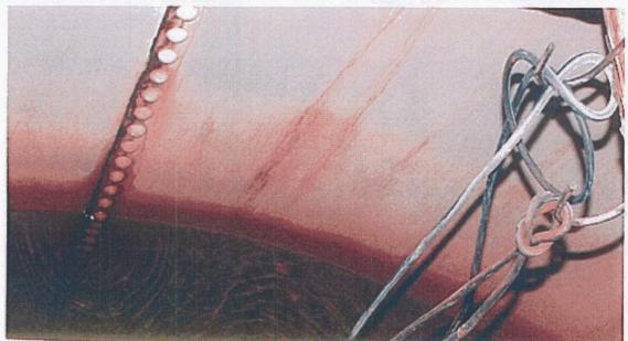
Photos show the condition of the interior liner. We recommend sandblasting all rusted and abraded areas of the tank interior to an SSPC #10 (near white) blast, brushblast all remaining areas, stripe coating all seams and welds, then applying an epoxy liner to achieve 8-10 mils of dry film thickness.
