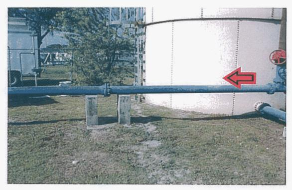
Photo shows the condition of the tank shell. The tank is not equipped with a manway. manway. The following items are required to bring tank in compliance with AWWA D100-96, section 7.1: Shell Manways, OSHA, and TSS, (see glossary pg. 8):
