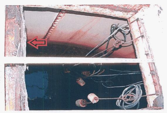
Photo shows the condition of the roof manway. Notice the manway curb is severely deteriorated. Roof openings on this tank require the following to be in compliance with OSHA, AWWA and TSS Section 7.0.8: Access, (see glossary pg. 23):
