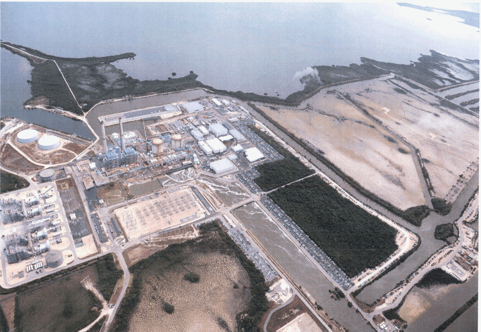
Docket No. 120009-EI Turkey Point Plant Pictures Exhibit TOJ-8, Page 3 of 5
