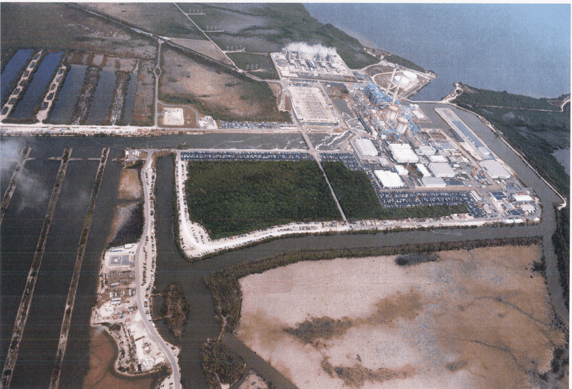
Docket No. 120009-EI Turkey Point Plant Pictures Exhibit TOJ-8, Page 2 of 5
