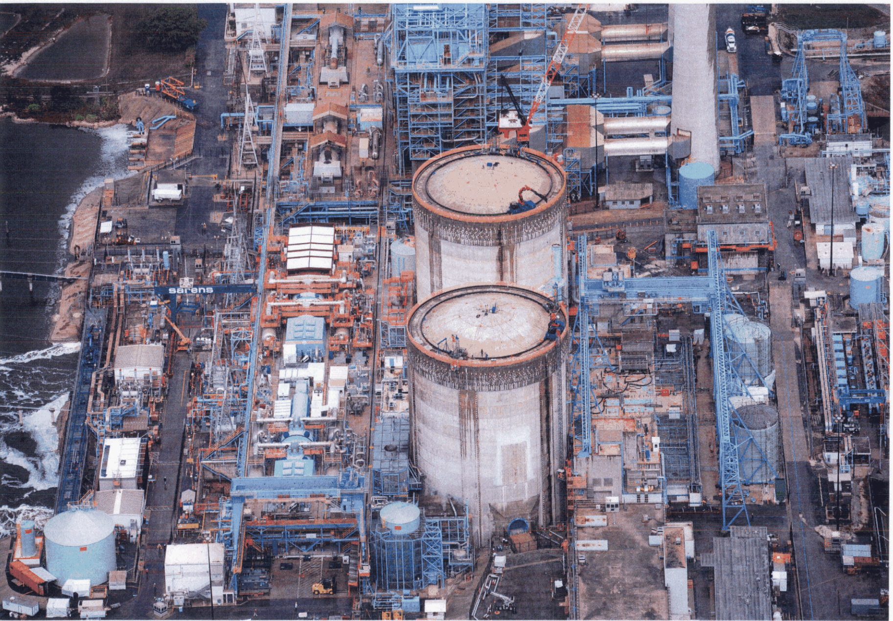
Docket No. 120009-EI Turkey Point Plant Pictures Exhibit TOJ-8, Page 5 of 5
