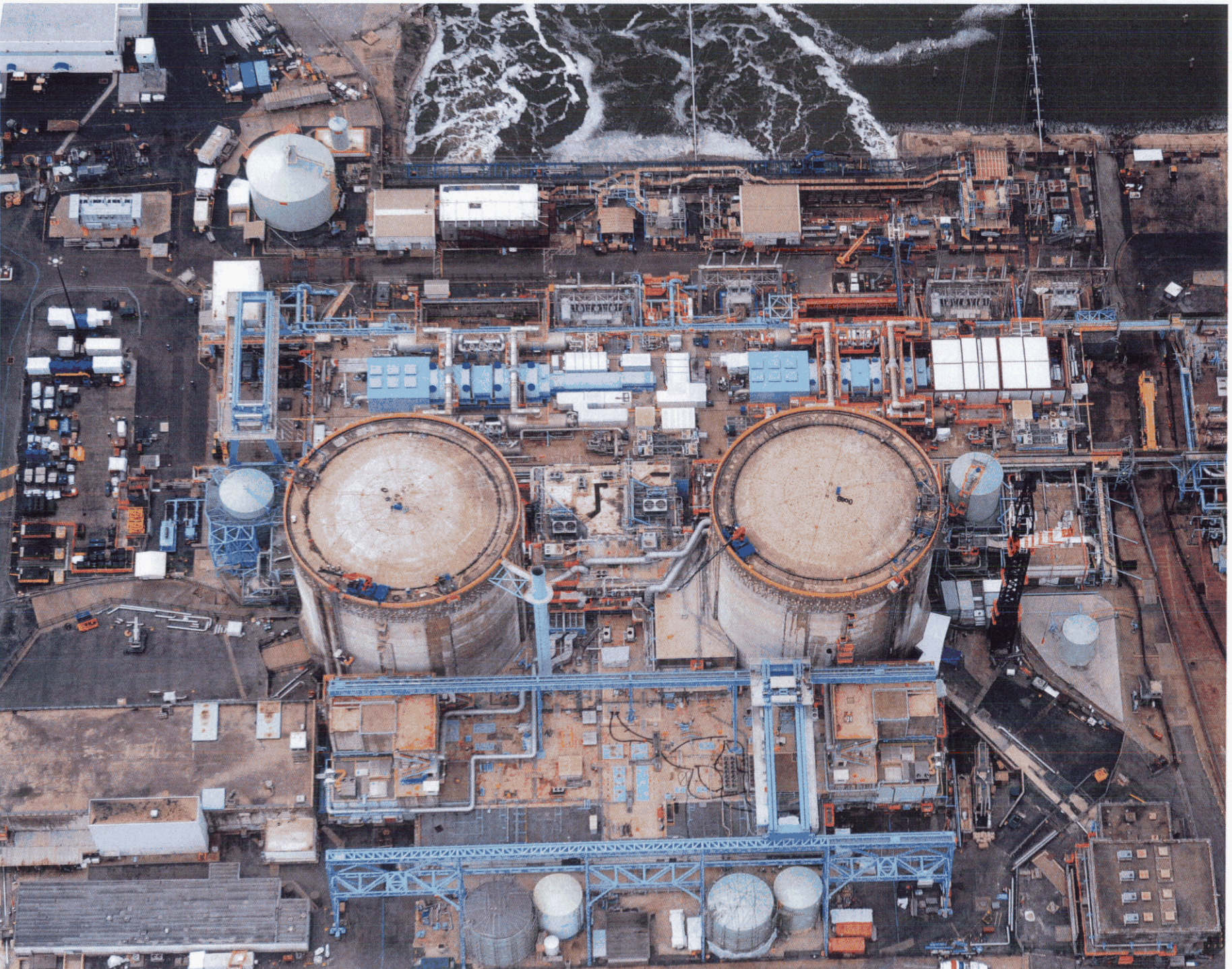
Docket No. 12009-EI Turkey Point Plant Pictures Exhibit TOJ-8, Page 4 of 5
