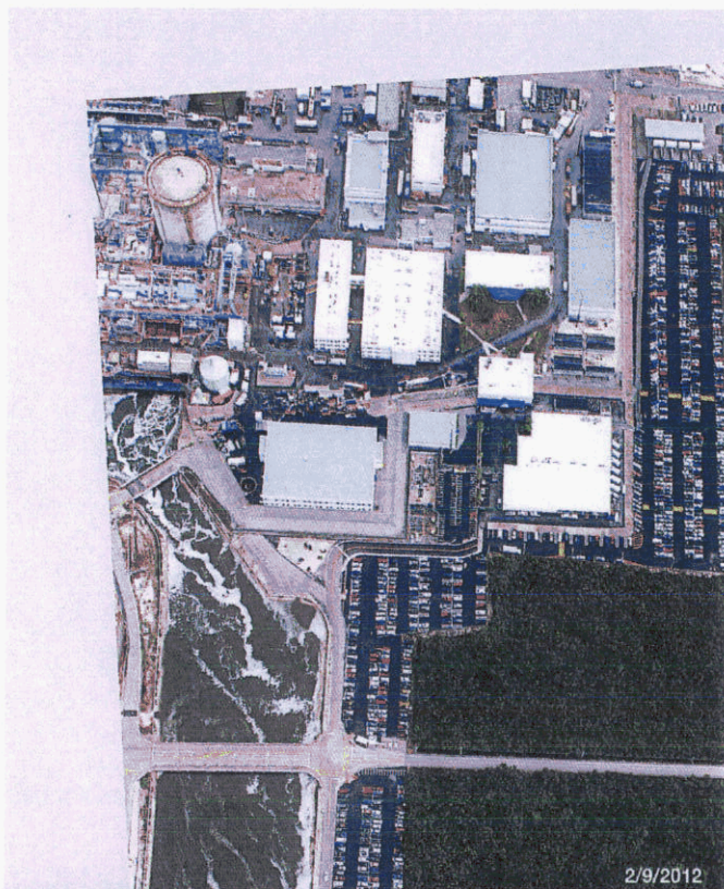
Aerial photo of Turkey Point plant during recent uprate activity depicts only a small portion of overflow parking for project workforce.
