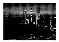
The station operates four (4) pulverized coal-fired steam units equipped with desulfurization scrubbers and electrostatic precipitators. The station's coal-fired units have recently undergone the addition of air pollution control systems called Selective Catalytic Reduction (SCR). The SCR installations occurred from 2007 to the spring of 2010. In addition, the station operates one (1) aero-derivative combustion turbine that entered into service in
