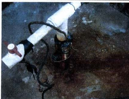
Water leaking around well head.
