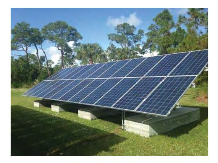
Strings in parallel: 2 Modules per string: 12 Total number of modules per array: 24<sup>°</sup> Max power rating for module@1000W/m2: 300 W Max capacity of the array:  $24 \times 300$  W = 7.2 kW
