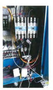
Figure 3 - Evaporator Fan Controllers
