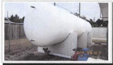
Hydro tank at Well #2
