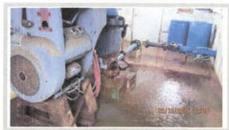
Leaking Well #2
