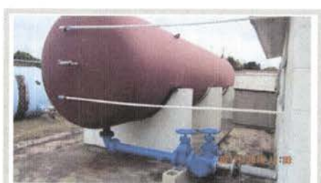
New Tank Well #4 (1/2016)
