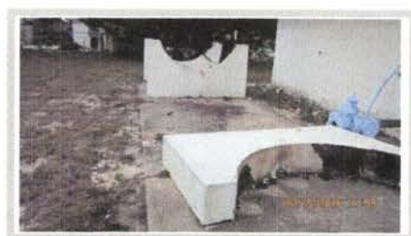
Former Tank Location Well #3
