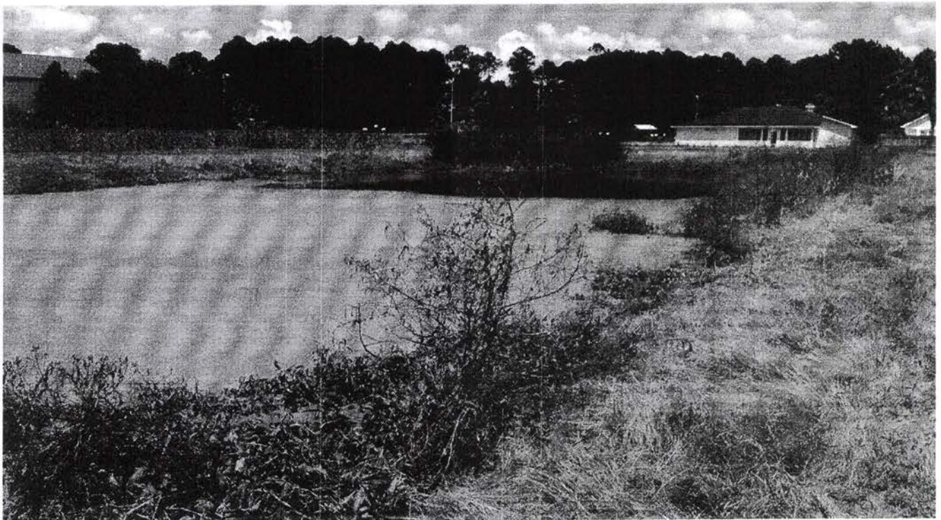
Figure 3: Percolation ponds were not being rotated in accordance with permit conditions. In addition, ponds were not being properly maintained; they were wet and overgrown.
