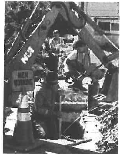
Service Upgrade: An Elizabethtown Gas Company crew – (from the rear) Mark Smith, Robert Crotty and Ruben Rivera – upgrade a service line to improve customer service.
