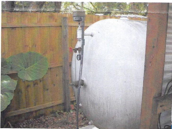
hydropneumatic tank
