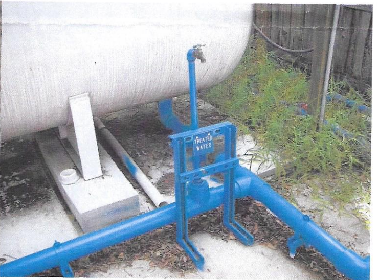
point of entry tap
