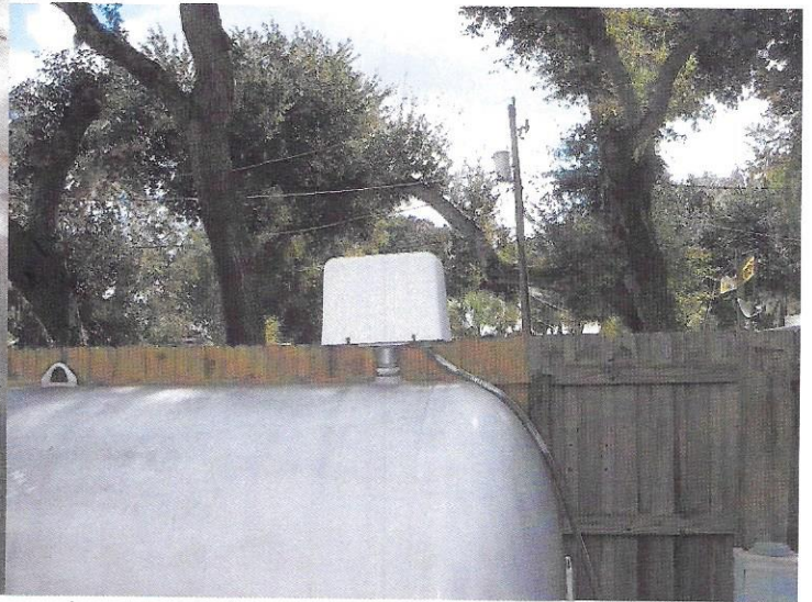
air compressor on tank
