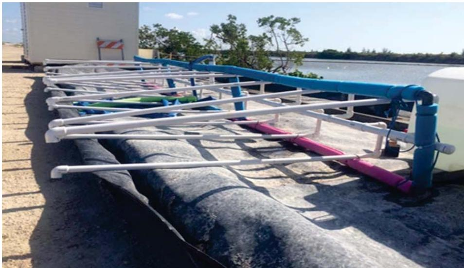
Figure C-2. Flocculent Injection Manifold (on its side)
