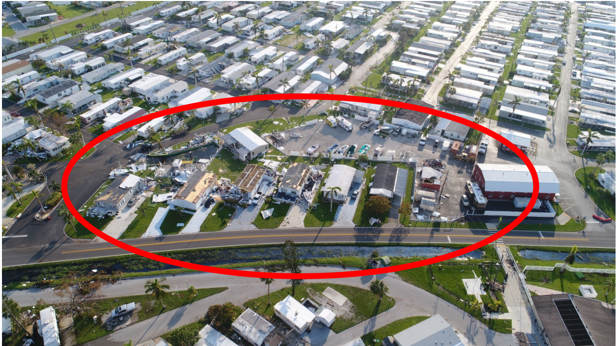
Area of concentrated damage, looking west.
