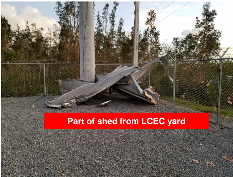
Belle Meade Substation (Looking West)
