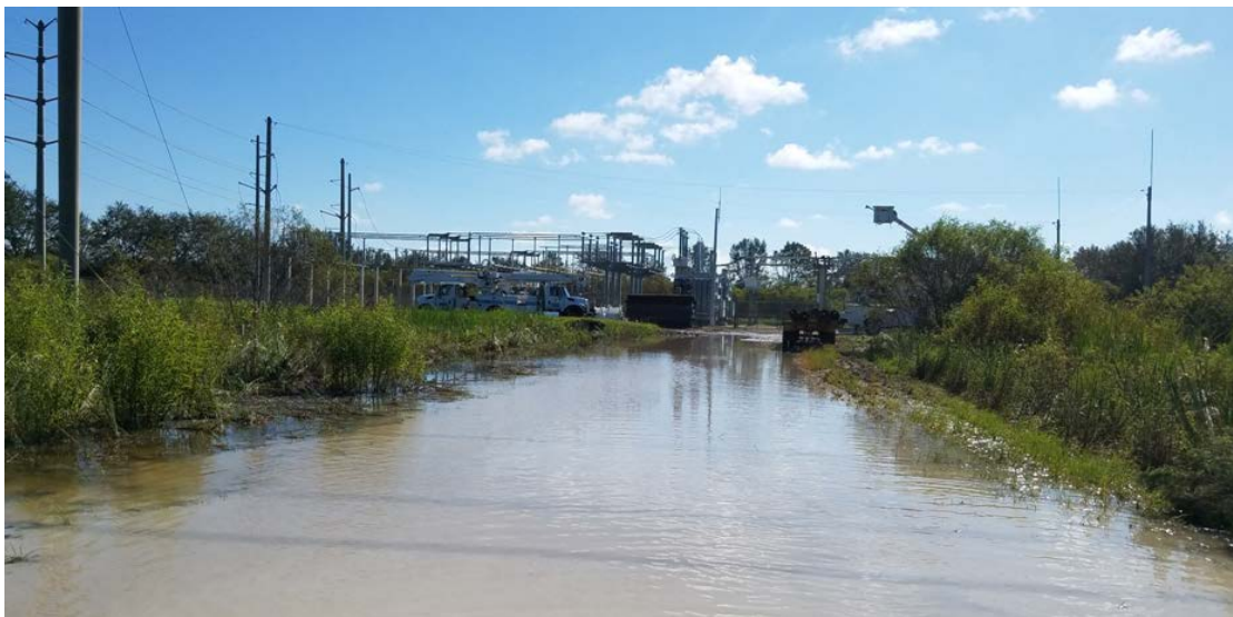
Corkscrew Access Drive
