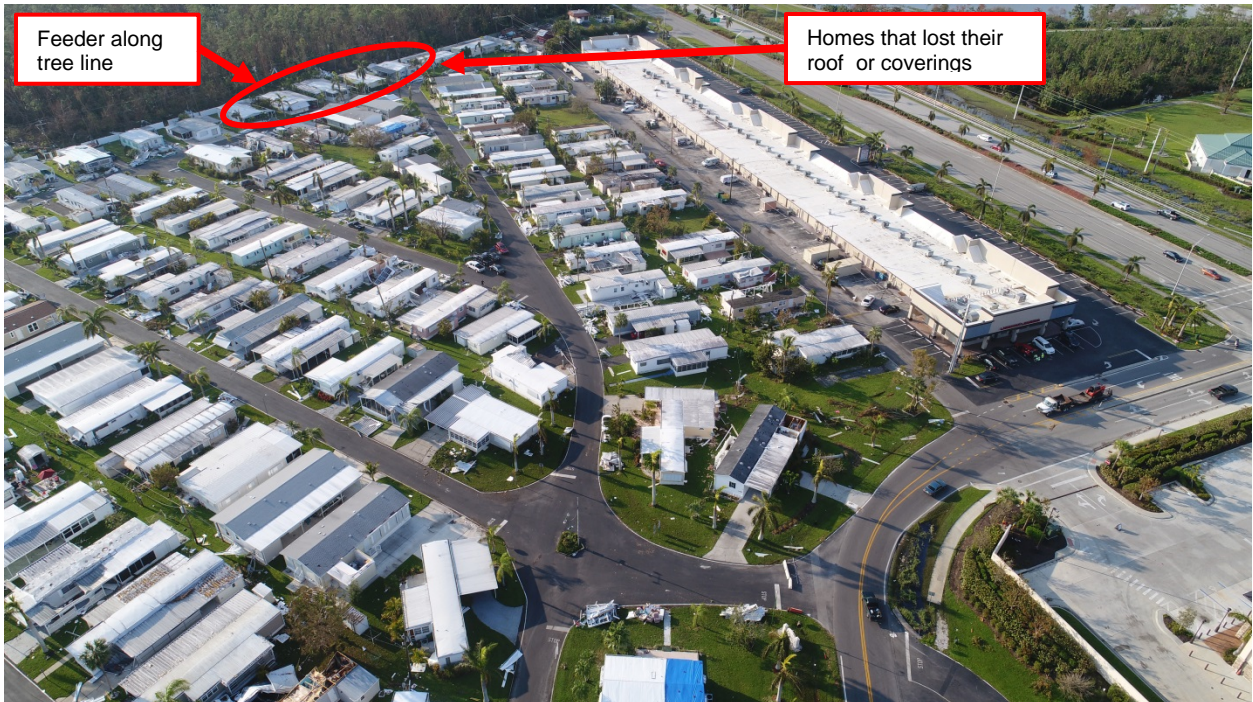
Looking northwest through the trailer park toward the feeder
