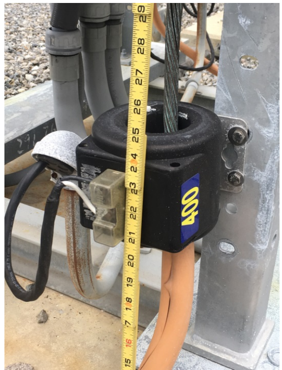
Fault bus CT's were submerged throughout entire substation
