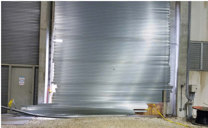
Watkins Substation – Overhead Door
