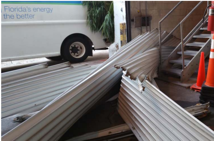
Watkins Substation – Overhead Door
