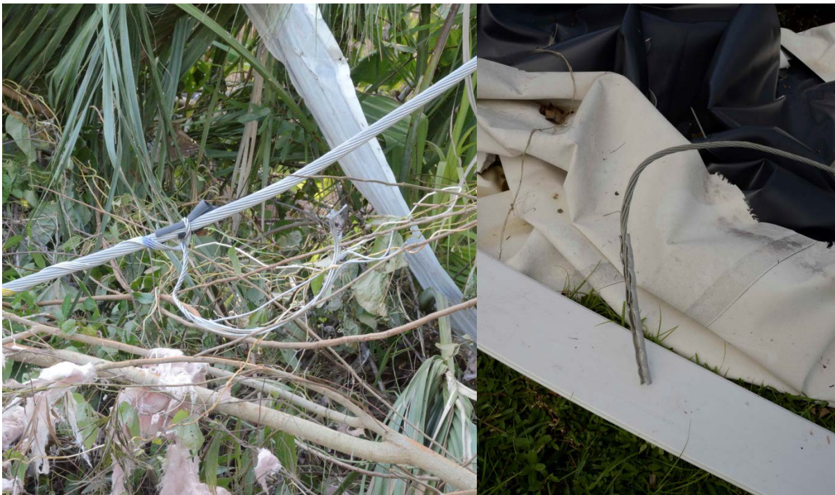
Insulator tie and failed splice. Below: ALS out of support and on ground
