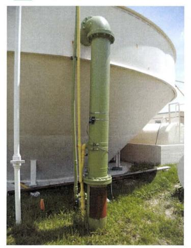
Figure 9. Corrosion on manifold pipe leading to Accelator.
