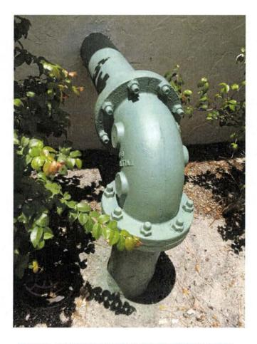
FIGURE 4. CORROSION ON FLUSH-LINE WELL #1. FITTING TIGHTENED, WIRE BRUSHED, ANTI CORROSION COATED.
