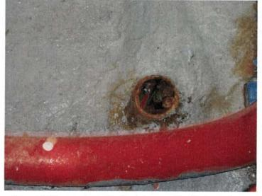
Figure 13. Exposed electrical wiring near the high service pumps. This is not found as a deficiency because they are not electrically active and the conduit is plugged; however, it is recommended to cap or otherwise cover the exposed wires.
