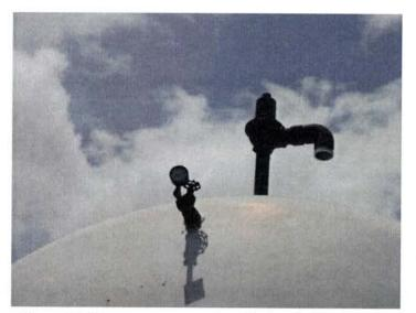
Figure 15. New pressure gauge installed on hydro tank.
