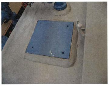
Figure 2. A plate with four (4) small holes was observed on top of the clearwell.
