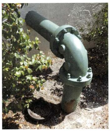
Figure 3. Corrosion observed on pipe leading from pump house for well#1.
