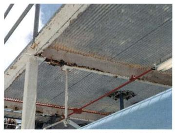
Figure 12. Corrosion on underside of walkway leading to Accelator.
