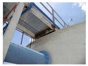
Figure 11. Corrosion on the underside of walkway leading to Accelator.
