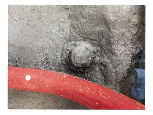
FIGURE 13. HS PUMP #2 DEAD WIRES IN ABANDONED CONDUIT SEALED & COATED.
