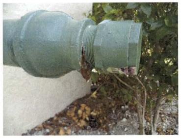
Figure 4. Corrosion and leak observed at the flush-line cap for well#1.
