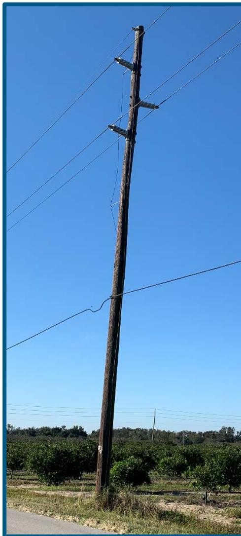
*Figure 1: Wood Pole to Non-Wood Upgrade candidate*
