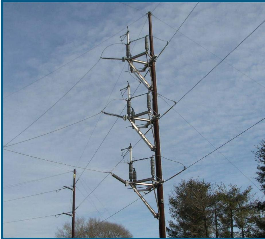
*Figure 3: DEF Manually Operated Switch*
