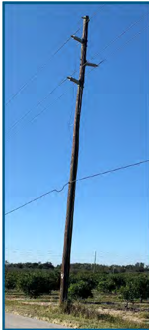
Figure 1: Wood Pole to Non-Wood Upgrade candidate
