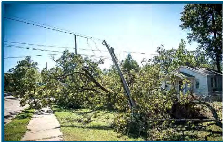
Figure 1: An example of residential customers that would be candidates for Undergrounding due to section of line and service in heavily vegetated areas.
