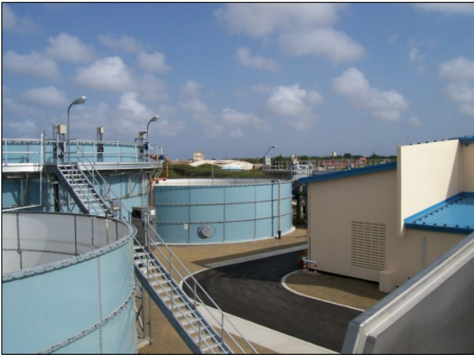
SBR Treatment Units
