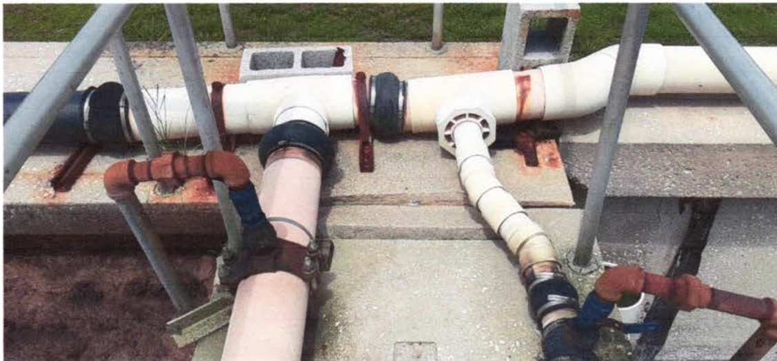
Item No. 2 of Deferred Maintenance Request Compressed air distribution lines have multiple temporary repairs that need to be repaired/replaced.
