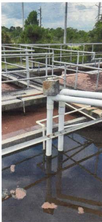
Item Nos. 4 & 5 of Deferred Maintenance Request The RAS/WAS collection box lines need replacement to support the RAS lines. (3 each 3" angle iron horizontal supports like the one pictured above) (3" angle iron vertical supports for the RAS/WAS collection box)
