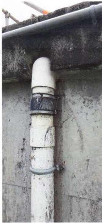
Item No. 6 of Deferred Maintenance Request The force main connecting to the WWTP from the master lift station needs repaired/replaced and sealed to prevent accidental discharge.
