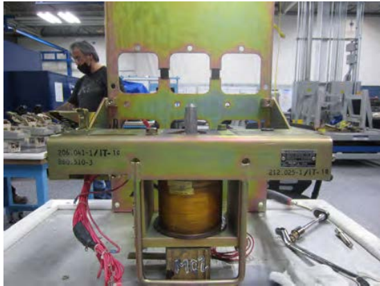
Phase 'C' Removed
