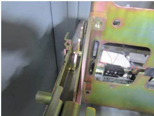
Breaker Frame Located in the Disconnect Position Stop Bracket
