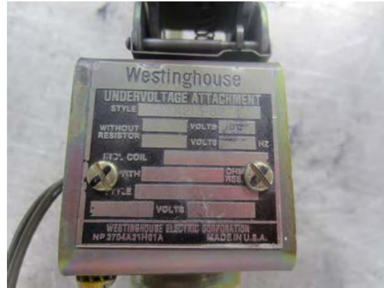
UVTA Assembly Removed
