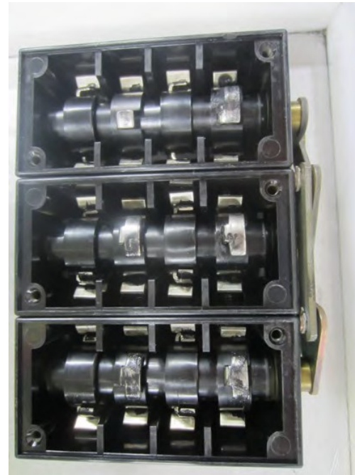
Rear of Auxiliary Switches
