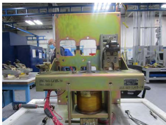
Phase 'B' Removed
