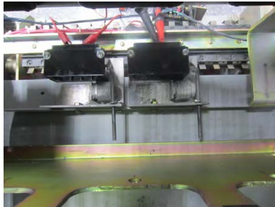
Breaker Frame Located in the Test Position Stop Bracket
