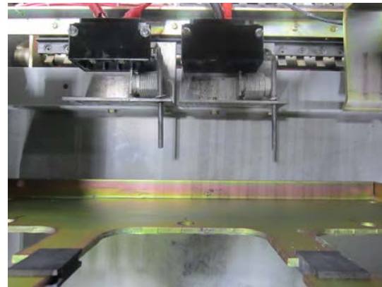
Breaker Frame Located in the Disconnect Position Stop Bracket
