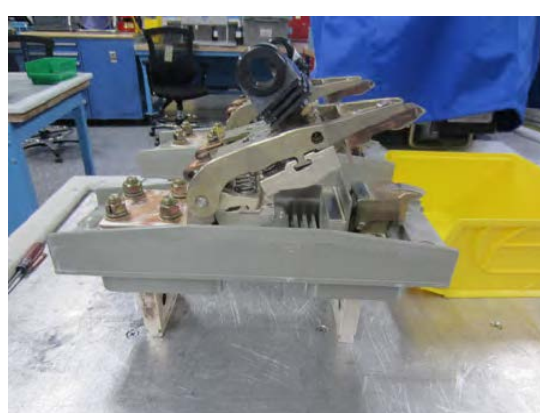
Phase 'B' Removed
