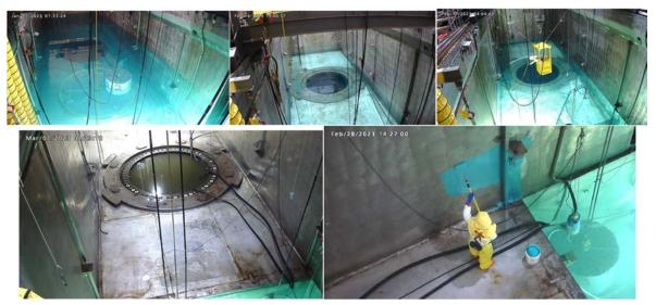
**Reactor Vessel Seal Plate**
