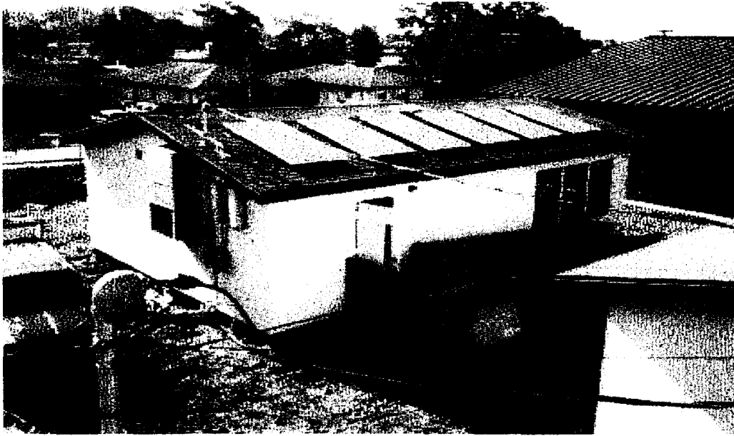
Figure 4-2 Portable Classroom Topped by PV Panels
