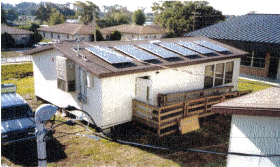
Figure 4-2 Portable Classroom Topped by PV Panels
