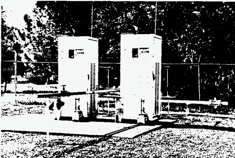
2nd Housing Area Vaporizers & Regulators
