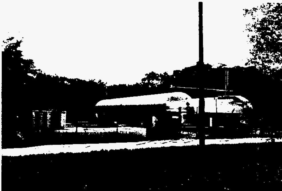
1st Housing Area 2-30,000 gal. Tanks
