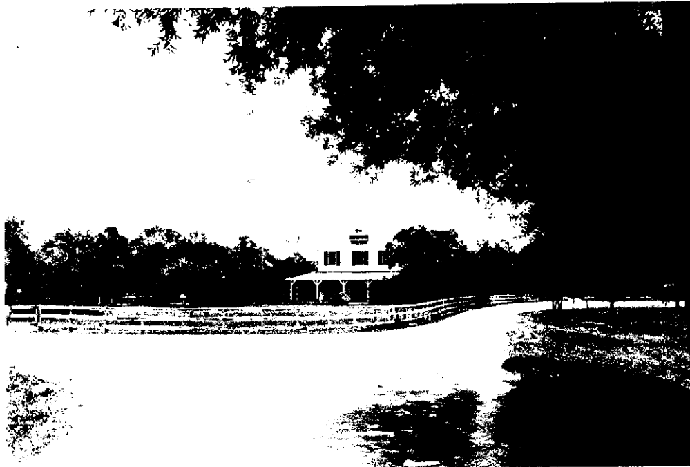
Close-up of Headquarters office.
