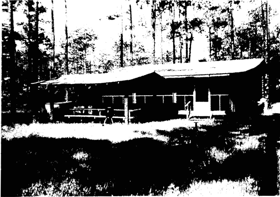
View of typical recreational lodging facility. This is RF-9 that is used primarily by the Ranch employees.
