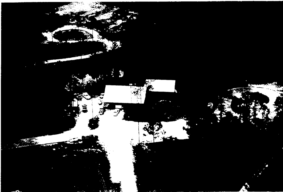
Close-up of Office Complex – View southeast
