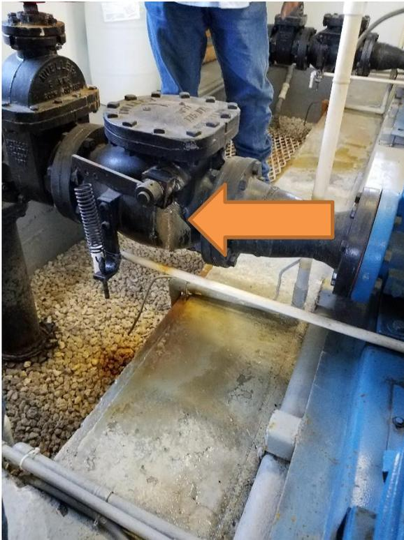
Photo 3: Arrow pointing to leak on valve on HS Pump-to be replaced soon per operator
