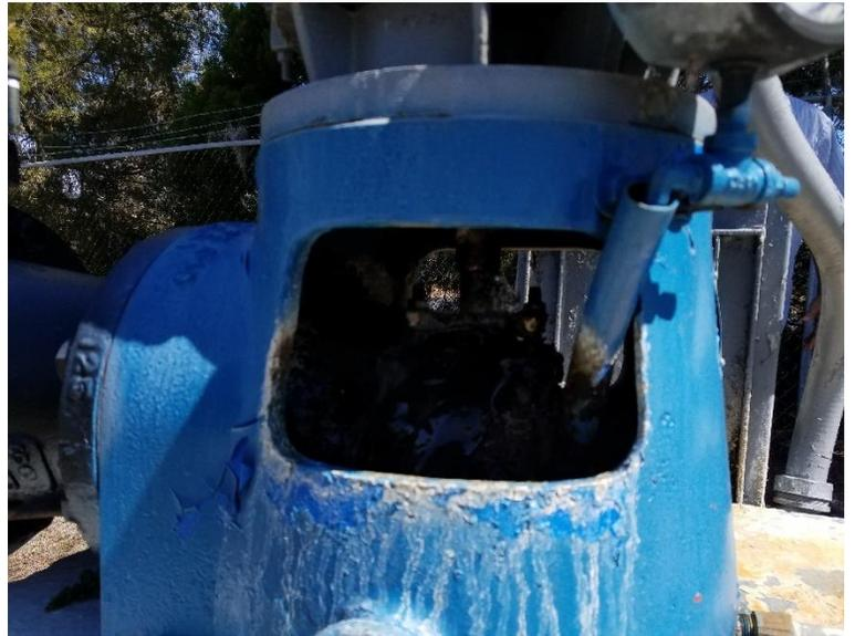
Photo 4: Excessive leaking on packing gland on well #1.
