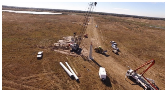
Typical Installation of a steel pole base
