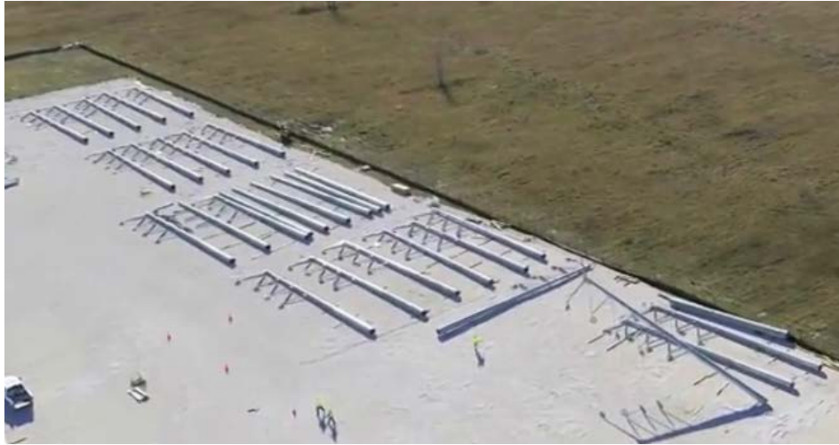
Framing the tops in the staging area
