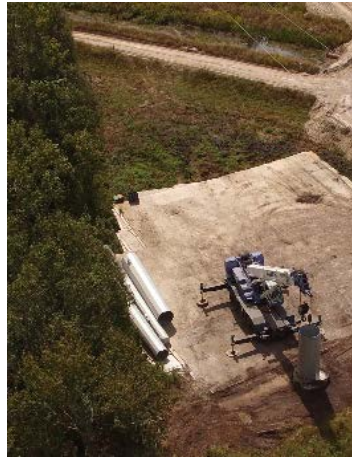
Example of a Base, Mid and Top staged at a proposed pole location
