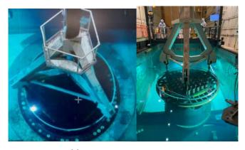
Lift and Transfer Core Support Assembly
