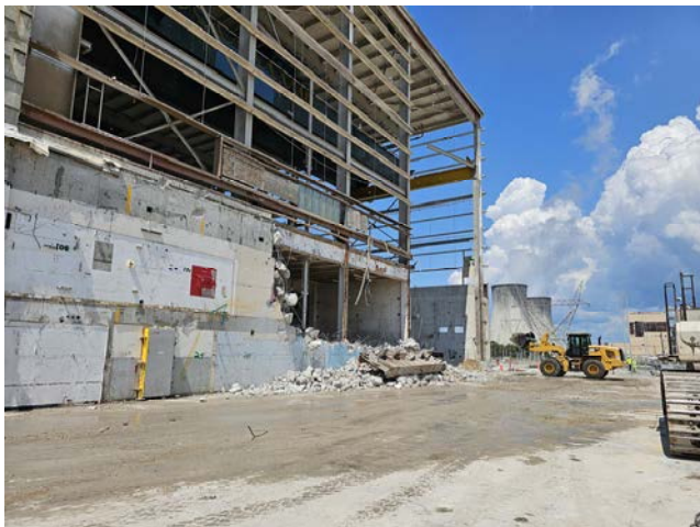
Turbine Building Demolition
