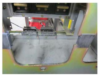
Cell Switches shown through Breaker Rear Panel
