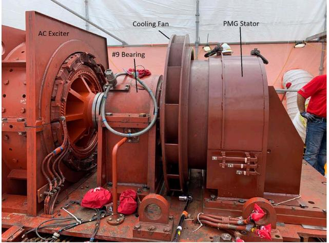
Fig. 2 U4 Exciter with PMG Stator Installed
