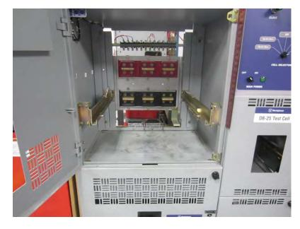
Left-Side Switch and Right-Side Switch Installed in Test Cell
