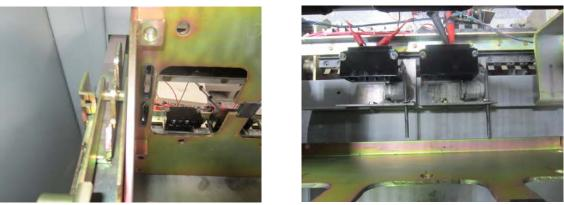
Breaker Frame Located in the Test Position Stop Bracket
