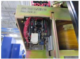
Control Relay with Front Cover Removed
