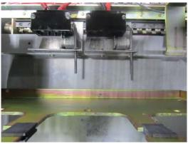
Breaker Frame Located in the Disconnect Position Stop Bracket
