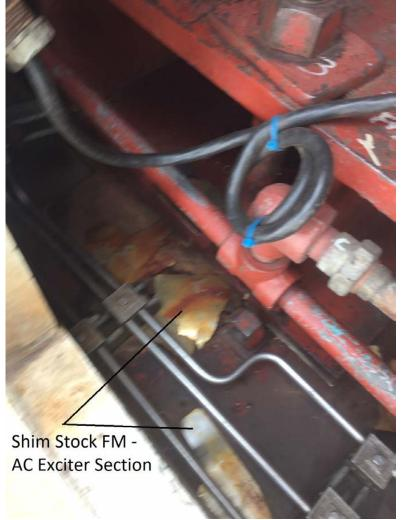
Fig. 11 Foreign Material (Shims) Found in AC Exciter Section
