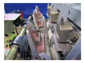
Breaker Open, With Arc Chutes Removed
