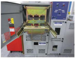
Breaker Frame on Test Cell Rails
