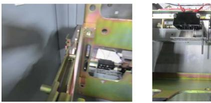
Breaker Frame Located before the Cell Positioning Stop Bracket
