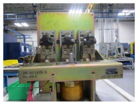
Breaker with the Operating Mechanism Removed
