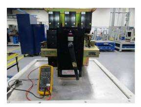
Breaker Closed, Switch Contact Open
