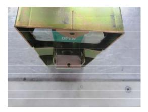
Bent Breaker Lock-Out Tabs
