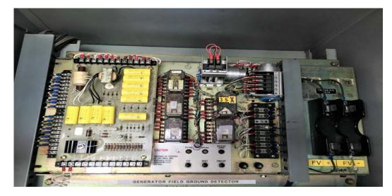
The ground detector panel provides an automatic ground check on the Generator rotor and exciter rotor once every 24-hours. Three push buttons switch are located on ground detector module for TEST- RESET – SIMULATE function with status indication lights. Operation of the test switch allows a ground check to be performed manually at any time.
