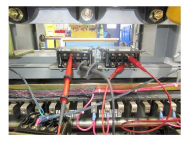
Cell Switch Monitoring Set-up
