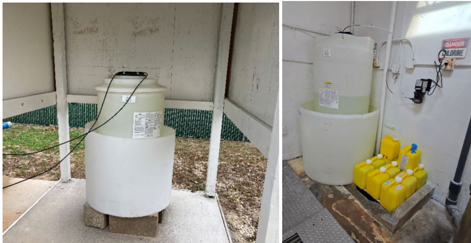
9 10 Liquid Chlorine Spill Containment Measures
