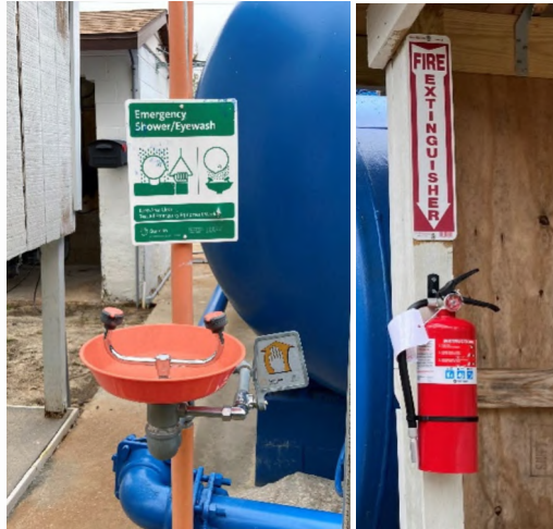
Emergency eye wash station (left), fire extinguisher (right).
