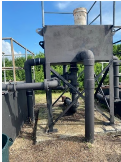
Figure 2-5: Flow Splitter Box
