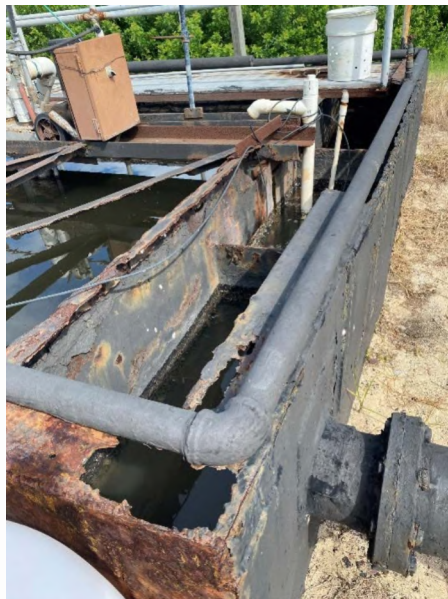
Figure 2-1: Plant 1 Corrosion and Rust
