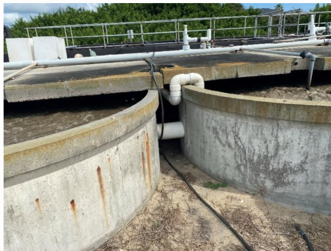
Figure 2-16: Plant 2 Aeration Basin Tanks & Piping
