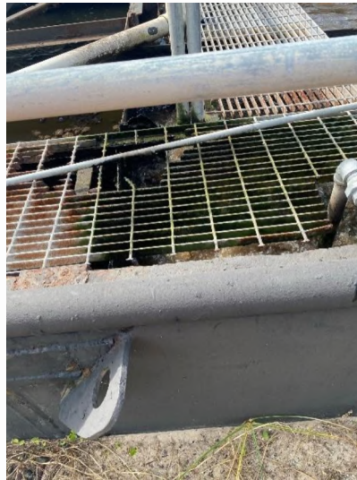
Figure 2-35: Structural Corrosion
