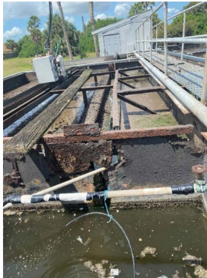
Figure 2-2: Plant 3 Corrosion and Rust
