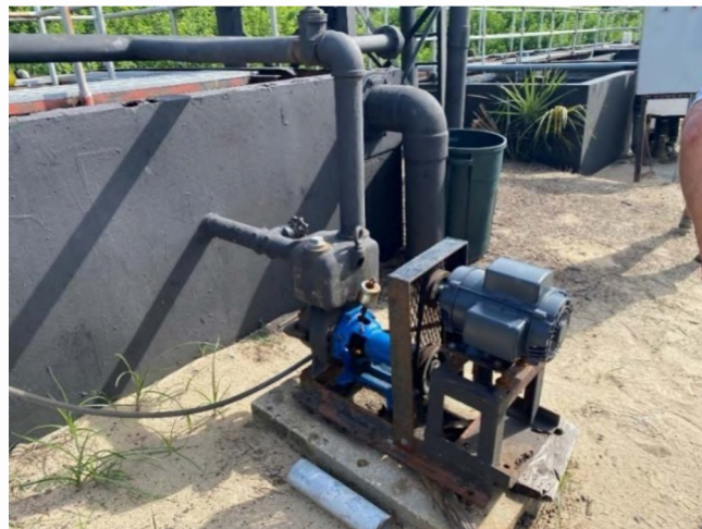
Figure 2-4: Surge Tank Pump
