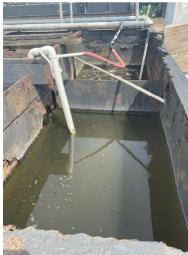
Figure 2-26: Plant 3 Chlorine Contact Chambers and Effluent
