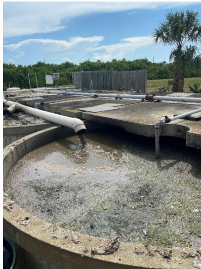
Figure 2-18: Plant 2 Aerobic Digester
