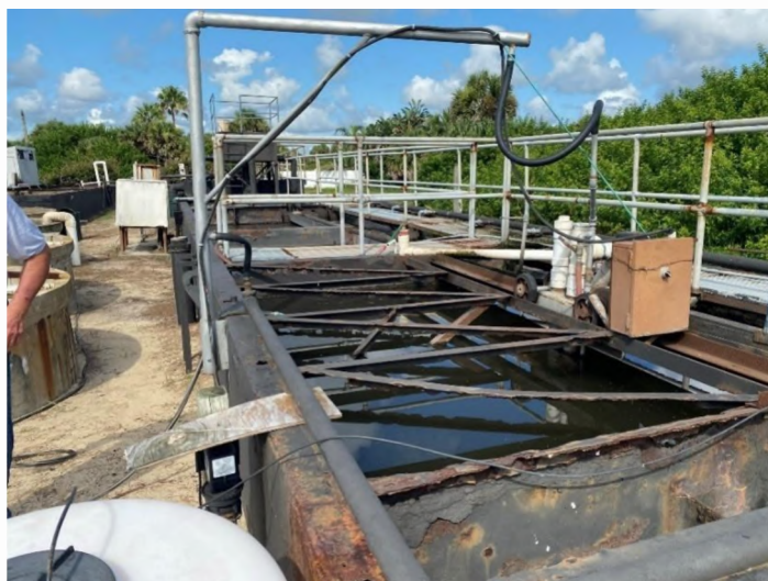
Figure 2-8: Plant 1 Clarifier
