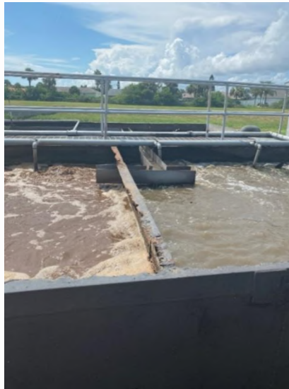
Figure 2-25: Plant 3 Stabilization Tank Chambers and Trough
