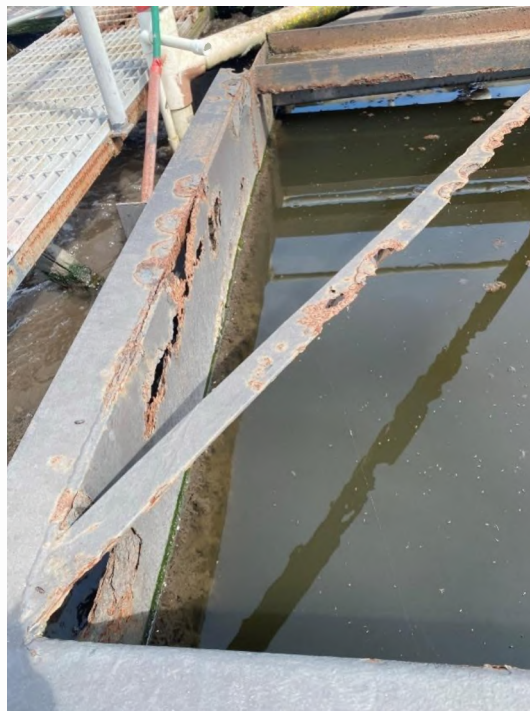
Figure 2-35: Structural Corrosion
