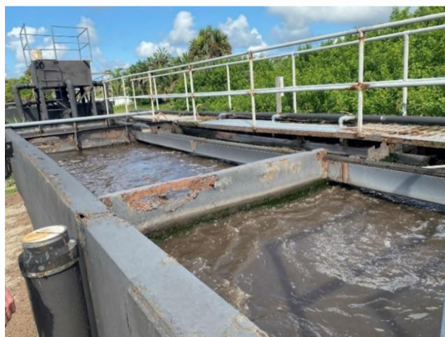
Figure 2-6: Plant 1 Aeration Basin
