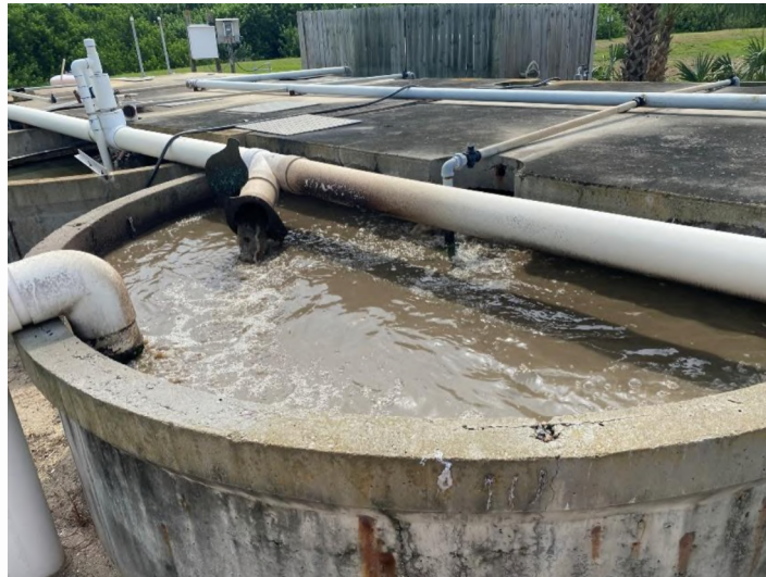
Figure 2-16: Plant 2 Aeration Basin Tanks & Piping
