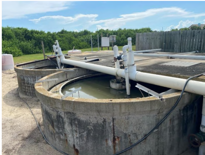
Figure 2-18: Plant 2 Aerobic Digester
