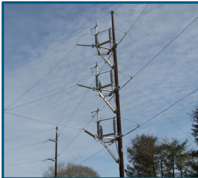
Figure 5: DEF Manually Operated Switch
