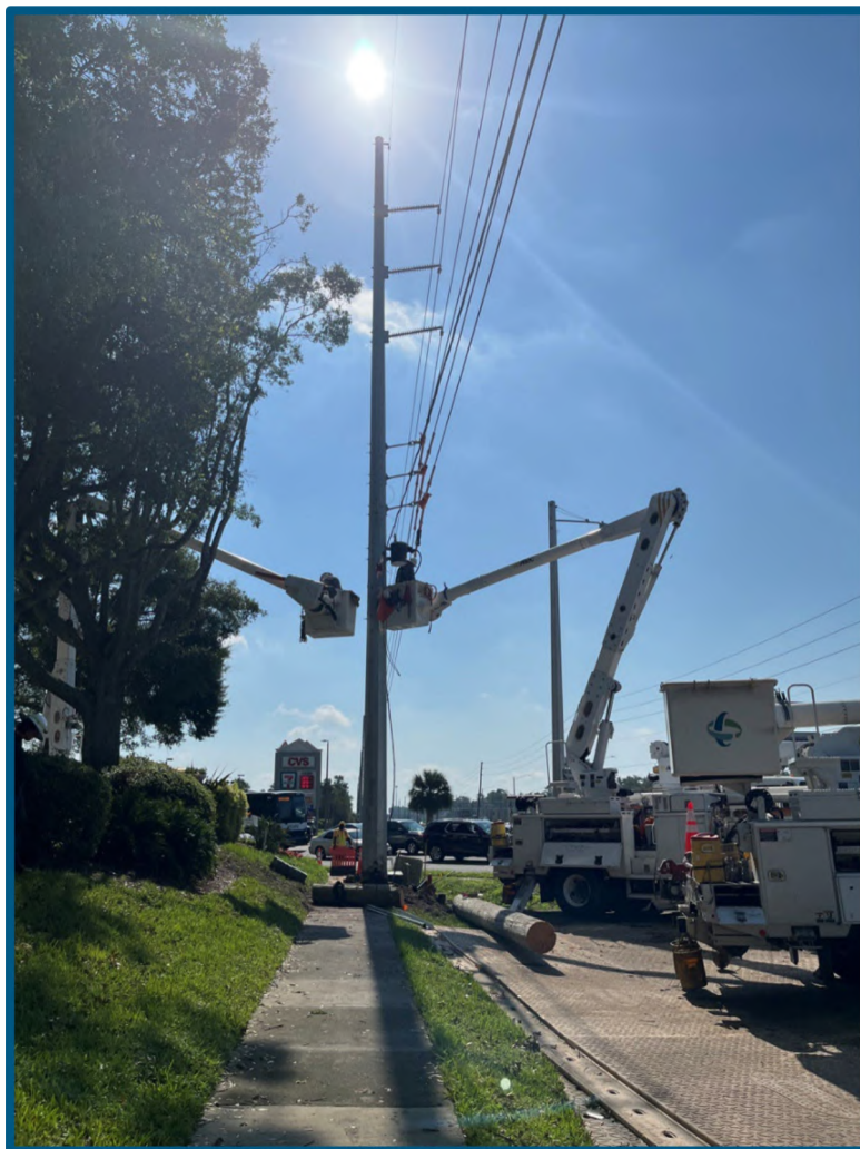
Figure 3: Wood to non-wood upgrade.
