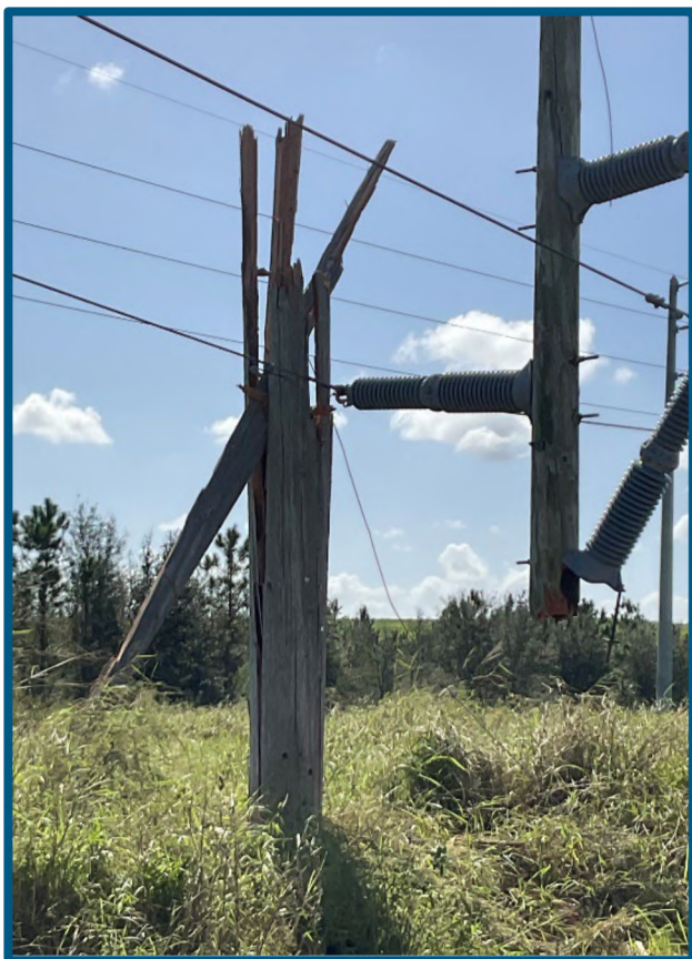
Figure 1: Broken Pole due to extreme weather event.
