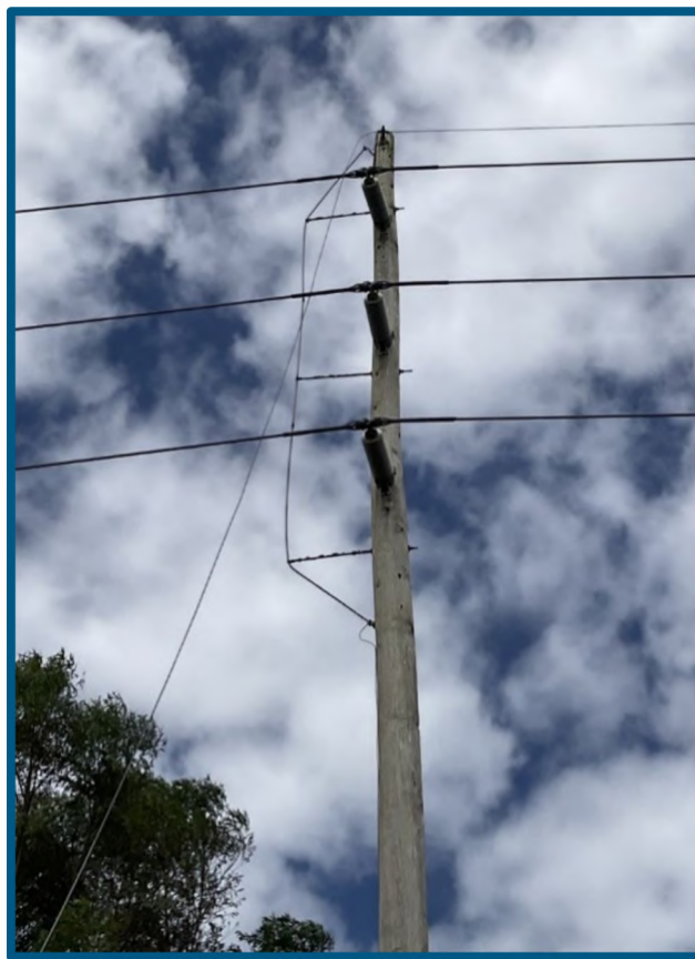
Figure 2: Broken Static due to extreme weather event.
