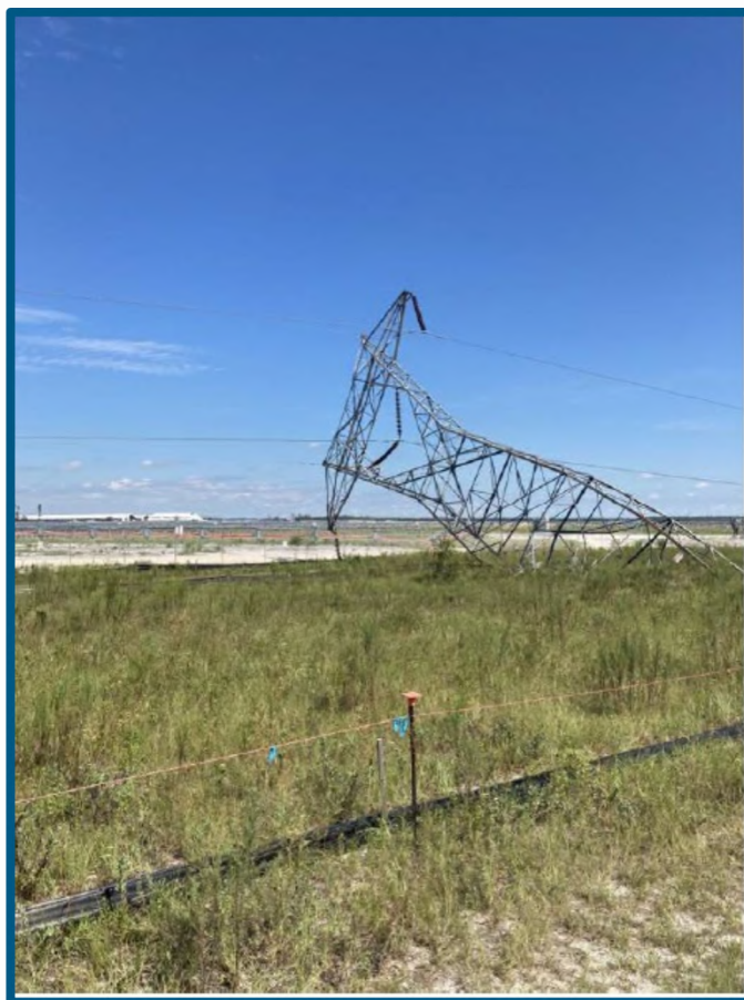
Figure 4: Lattice Tower impacted by Hurricane Idalia
