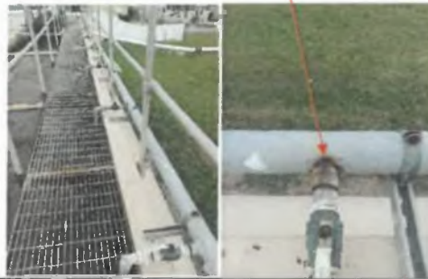
Leaking Piping
