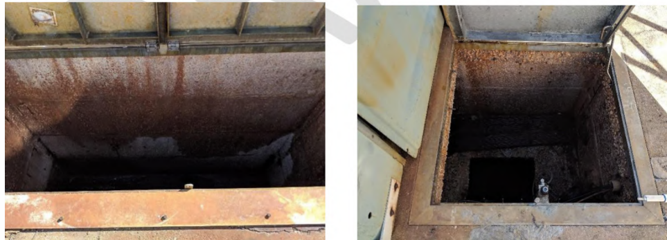
Figure 2: Existing Master Lift Station
