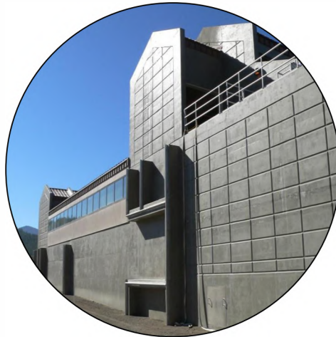
10 MGD Tahoe-Truckee SD BIOSTYR - Truckee, CA
