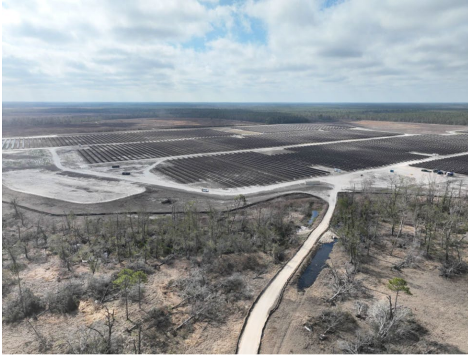
FIGURE 3.2 Sundance Solar Power Plant
