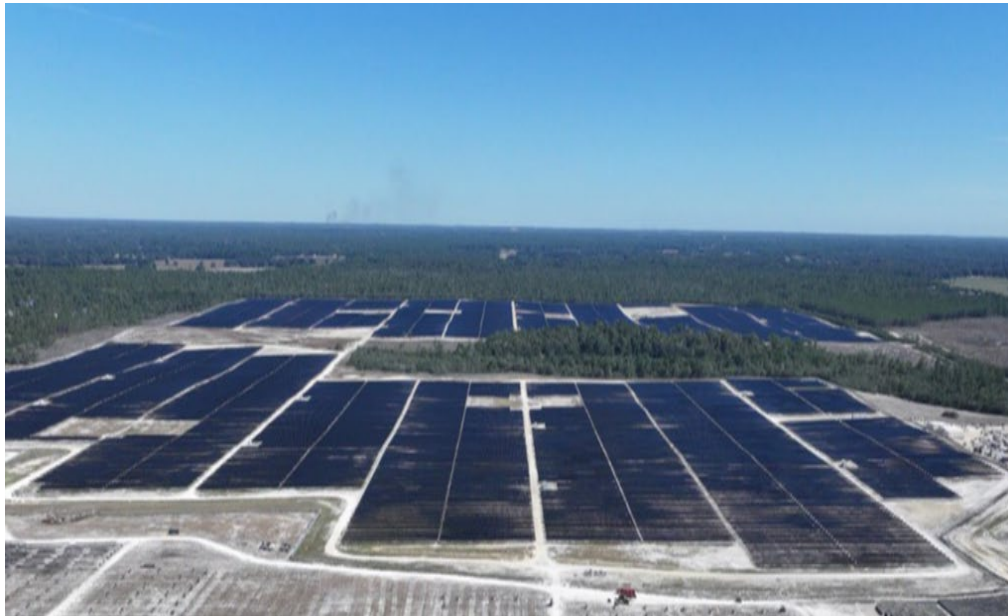
FIGURE 3.3 Half Moon Solar Power Plant
