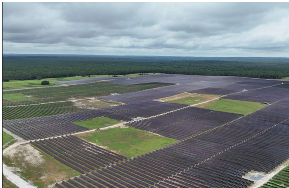
FIGURE 3.4 Rattler Solar Power Plant
