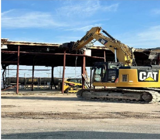
Receiving Warehouse Demolition
