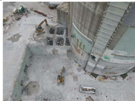
Seawater Room Roof Demo
