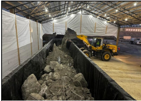
Loaded Rail Cars with Concrete Debris
