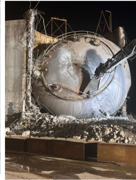
BWST- Steel Tank Demolition
