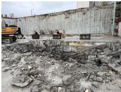
Decay Heat Vault Roof Demo
