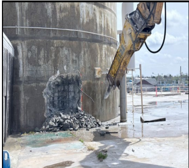
BWST- Creating a hole in preparation for RP Survey
