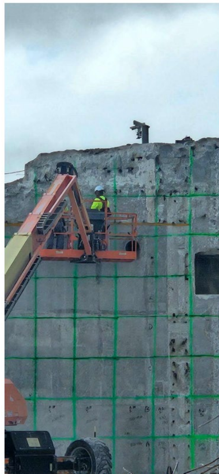
Scanning Auxiliary Building Wall
