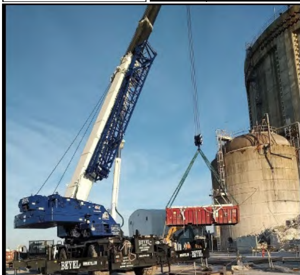
RB Phase 2 Internal Demo – Loadout at the Seawater Room
