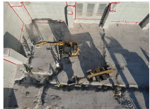
Turbine Building Drain Removal
