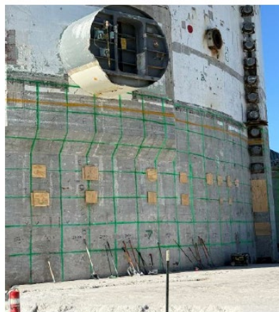
RB Exterior Wall Survey
