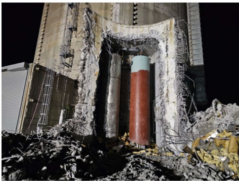
Building spray tank demo
