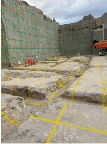
TB North and East Walls
