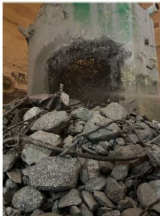
RB Core Barrel Removal
