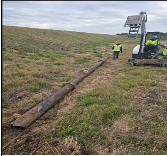
SDT-1 Buried Drain Line Removal
