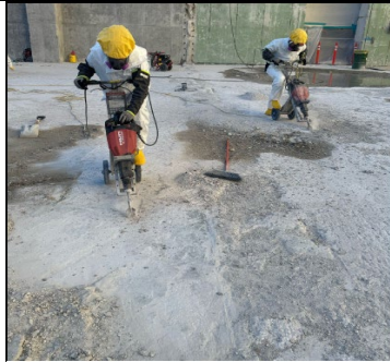
Power Block Final Decon – Floor Epoxy Removal
