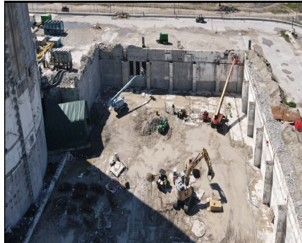
Power Block – Decon Wall paint Removal & RP Survey
