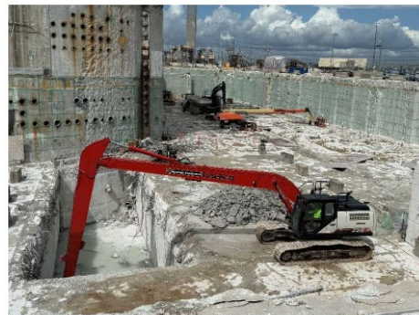
AB Decay Heat Vault Decon and Clean Out
