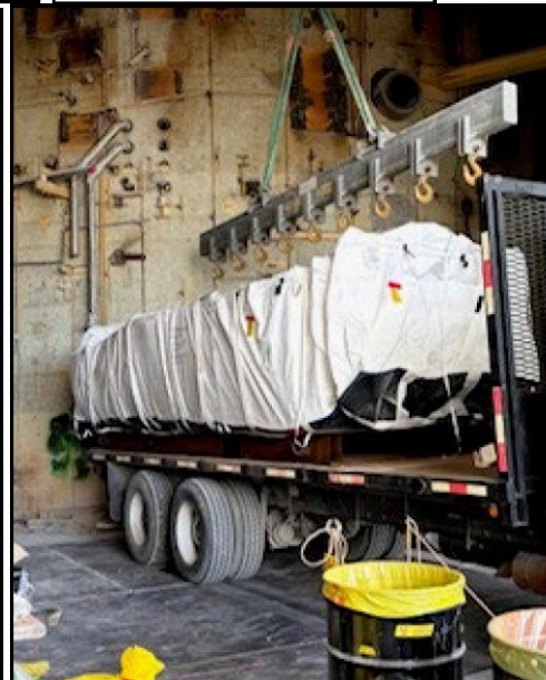
RB Phase 2 Internal Demo – Loadout
