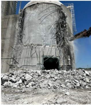
BWST- Concrete Removal
