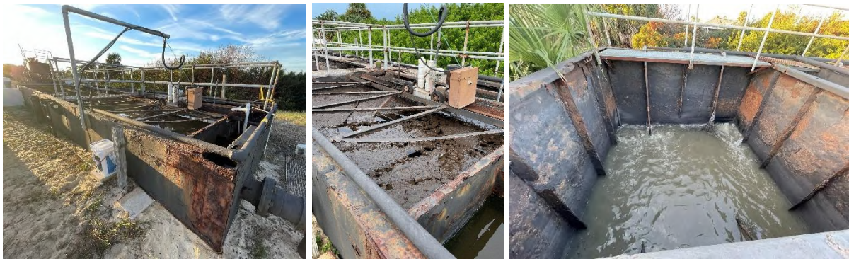
Examples of steel tanks and equipment deterioration at closing and examples of the numerous poorly installed welded patches on the tanks.
