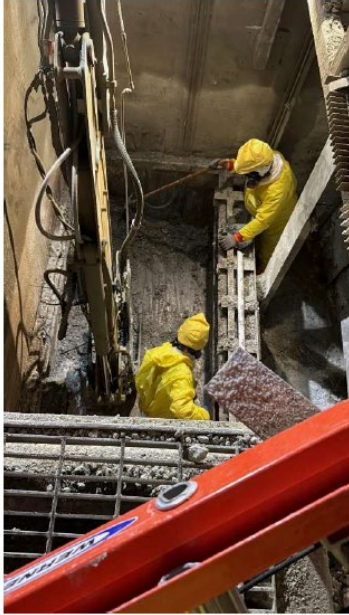
RB Sump Cleanout
