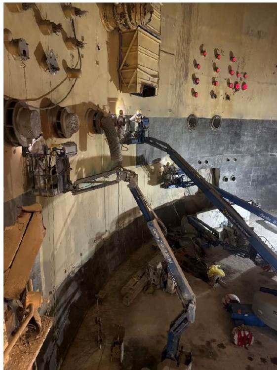
RB Paint Removal 95'
