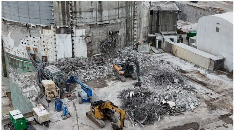
Intermediate Building Wall Demolition
