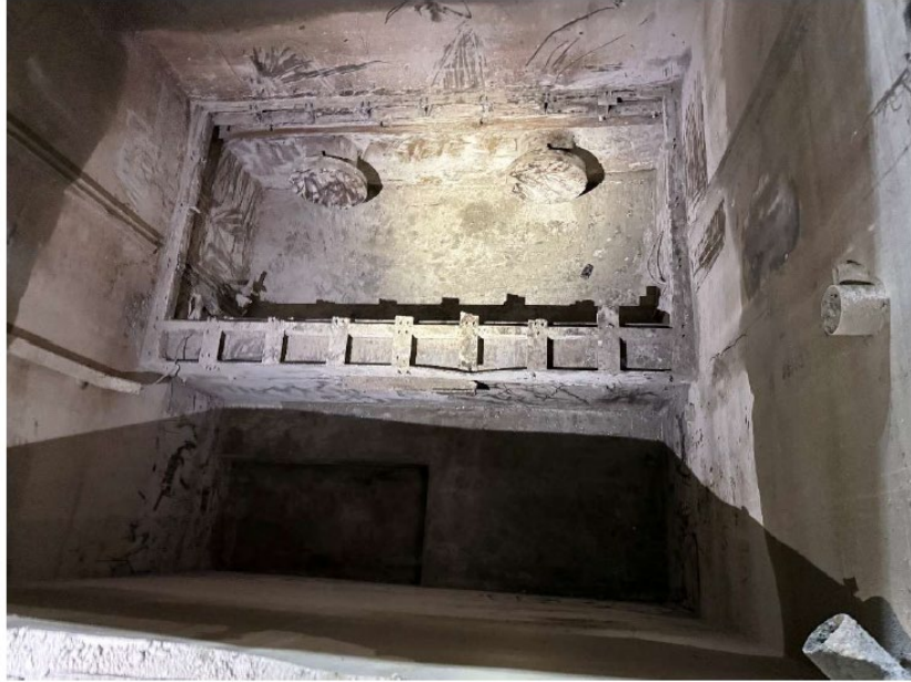
RB Sump Systems Removal
