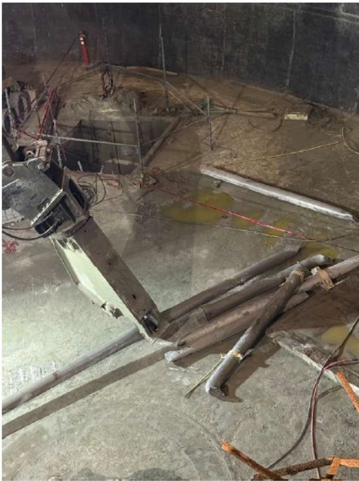
RB Building Spray Removal
