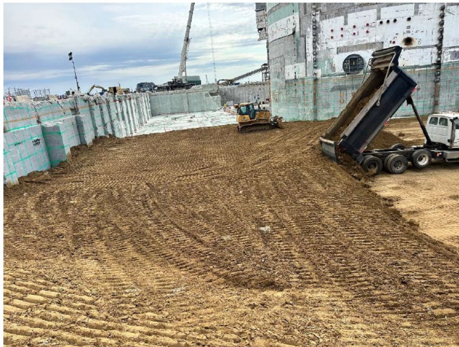
Turbine Building Backfill
