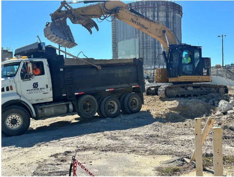
NAB Foundation Loadout
