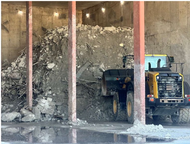
Mausoleum Material Loadout
