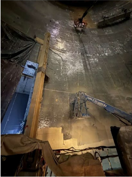
RB Paint Removal
