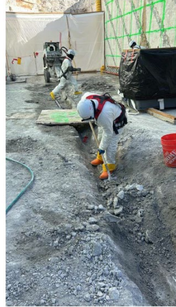
Decay Heat Vault Drain Removal
