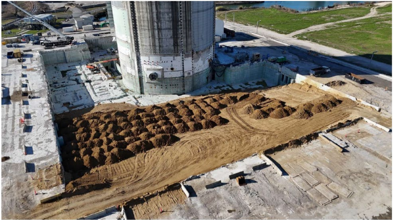
Turbine Building Backfill
