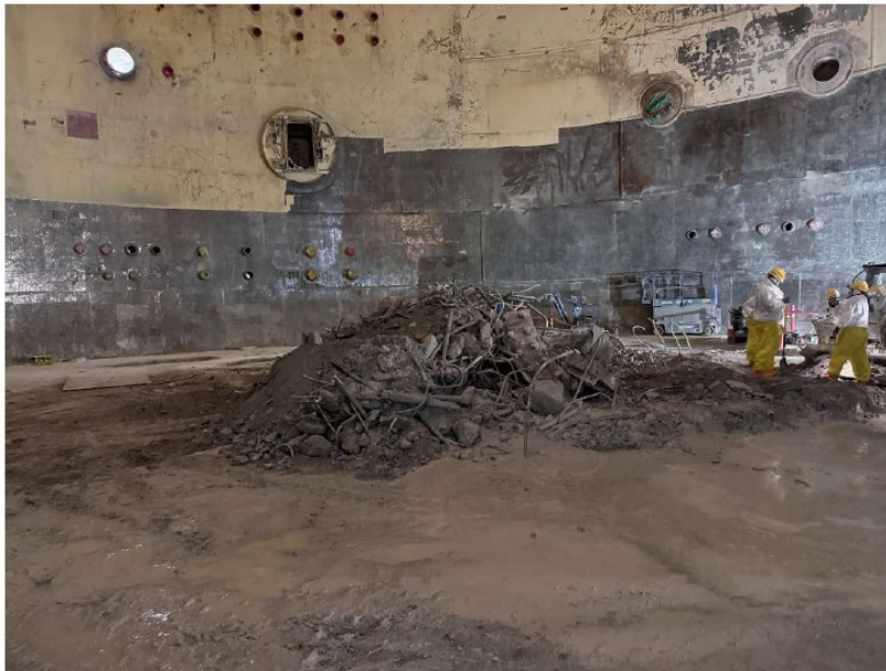
Reactor Vessel Support Loadout
