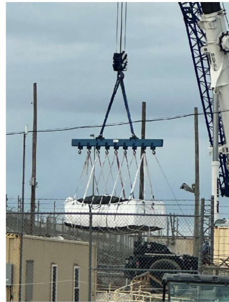
NAB Pad Loadout
