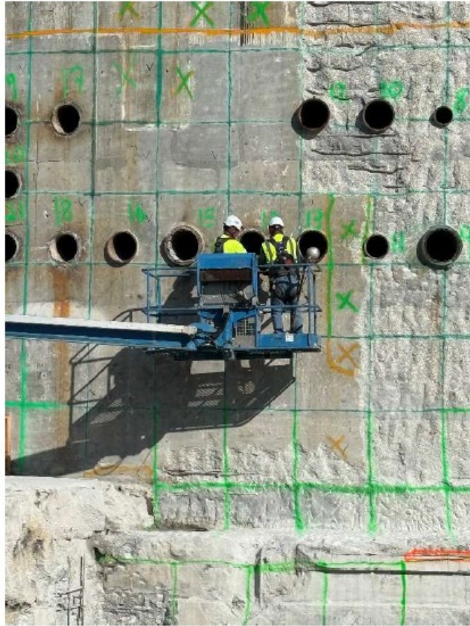
FSS Survey RB Penetrations
