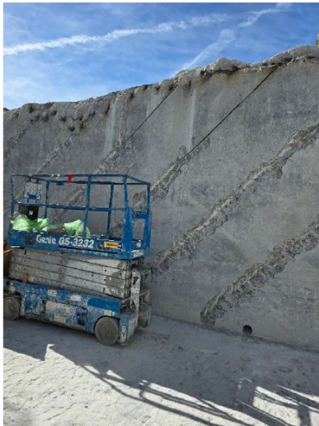
Decay Heat Vault Wall Remediation
