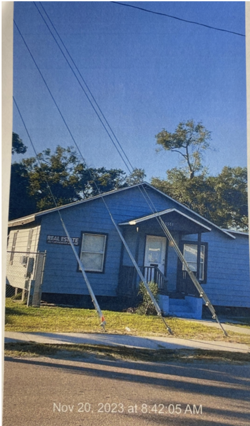
After Photograph-3 – Guy Wire Placement in front of Petitioner's Front Entrance
