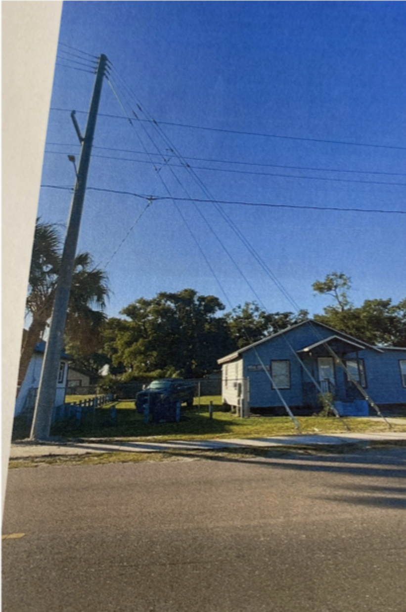
After Photograph-2 – Relocated Pole and Guy Wire Placement (Shows facilities relocated in front of Petitioner's front entrance)
