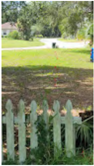
POWER LINE FROM POLE RISER SOUTH.jpg 2358K
