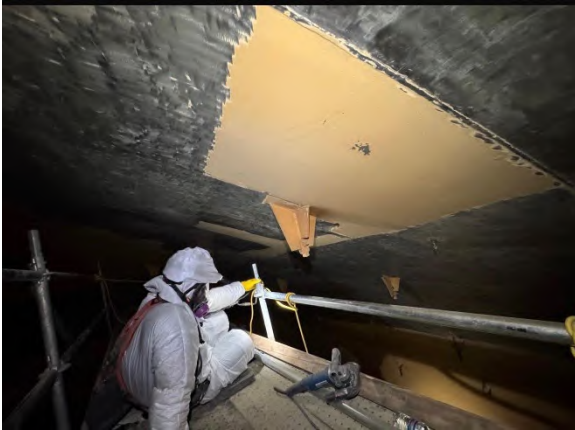
RB Dome Paint Removal
