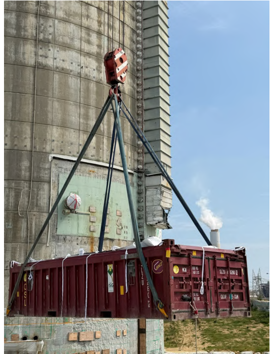
Intermodal Lifting from AB Basement
