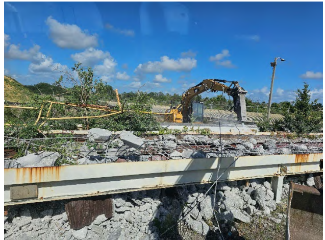
Hydrogen Farm Demolition
