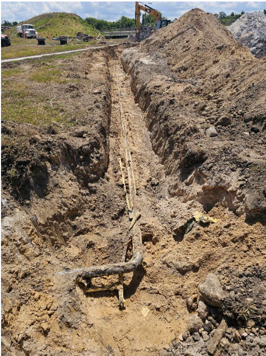
Hydrogen and Nitrogen Pipe Excavation
