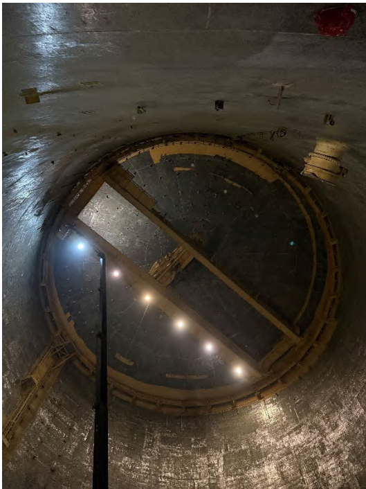
Paint Removal from 185' lift
