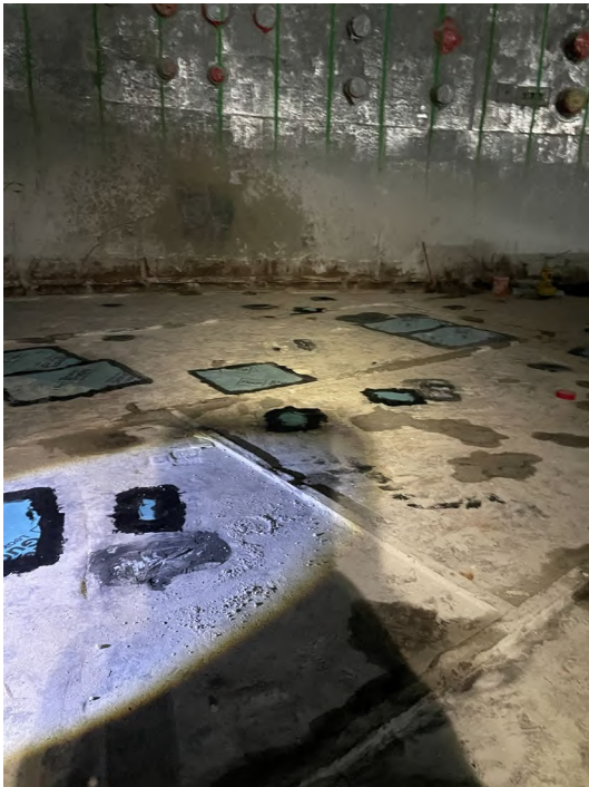
RB Subfloor Removal
