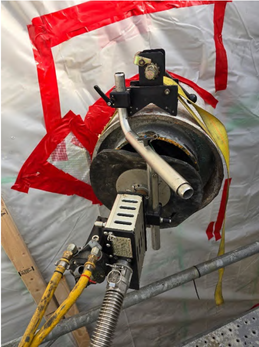
Hydrolazing Equipment Setup
