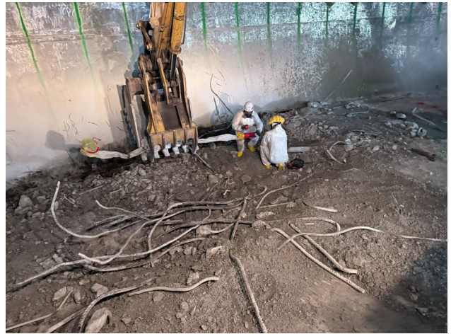
Floor Drain Removal
