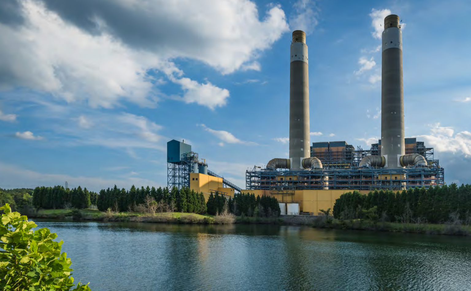
Belews Creek Steam Station
